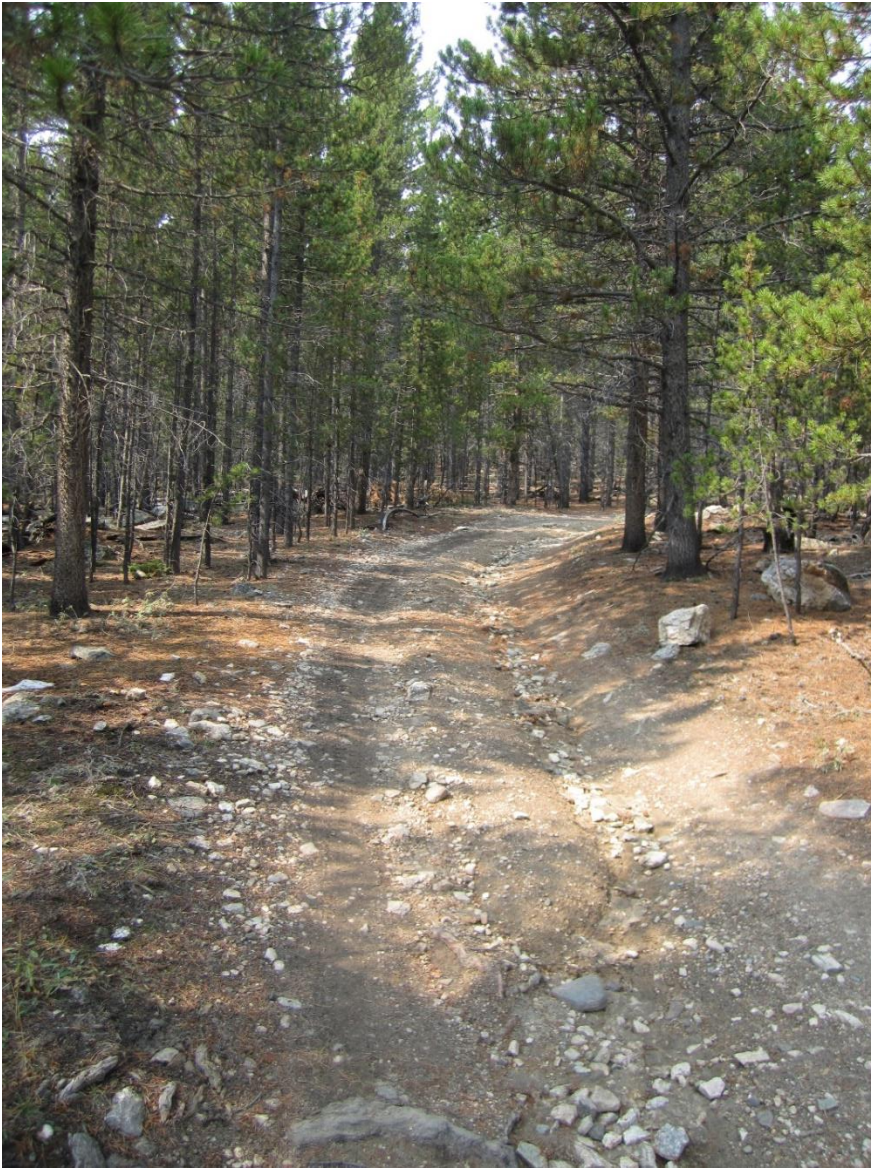
FDR 382 as a level 2 maintenance road with native surface. The entire length of FDR 382 used to be at this road maintenance level and should have remained at this level according to the BMW EA.
