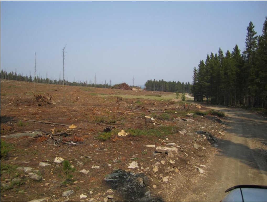
Unit 2C bordering FDR 382. This cut is part of the 370 acres of clear cuts for Unit 2a, 2b and 2c. Example of what the clear cuts look like.
