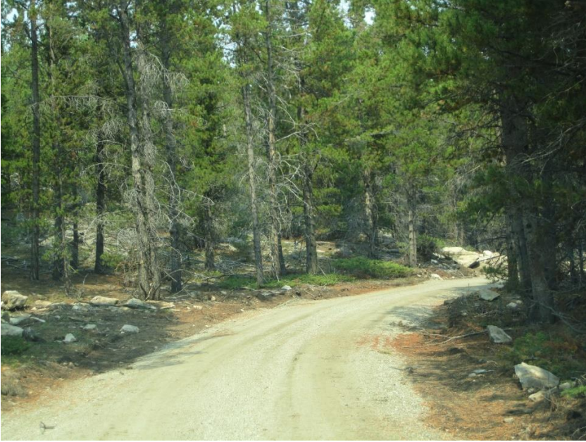
FDR 382 – Approximately 2.8 miles of the road is now surfaced. Travel time from US 16 to the CPW boundary now takes about 20 minutes versus the one-hour time before the road was surfaced. Surfacing was not authorized in the BMW EA. Road maintenance level upgraded from Level 2 to Level 3.
