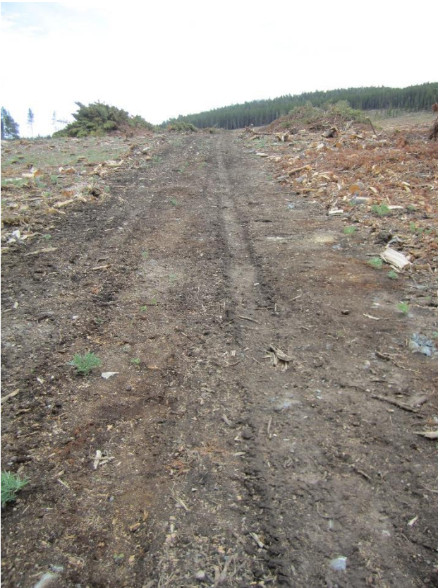
Temporary road not ripped to a depth of 8 inches. Not ripped at all. Vehicle tire tracks are the last use of this temporary road.
