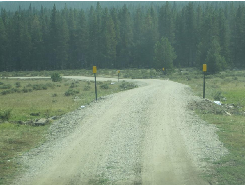
FDR 382 in Lynx Park. Note new culverts marked by the delineator posts. Culverts not needed for log trucks to remove timber.
